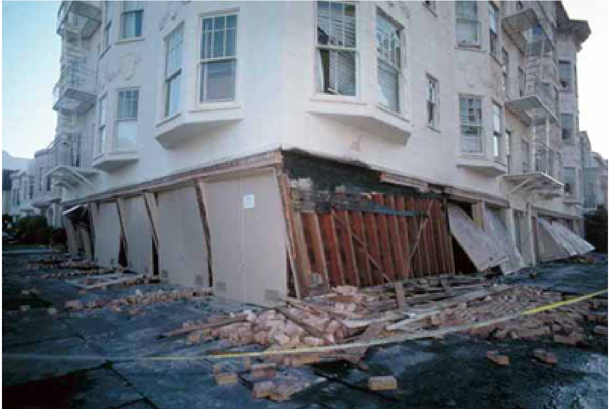
Figure 9-2. Soft-Story Damage from 1989 Loma Prieta Earthquake
