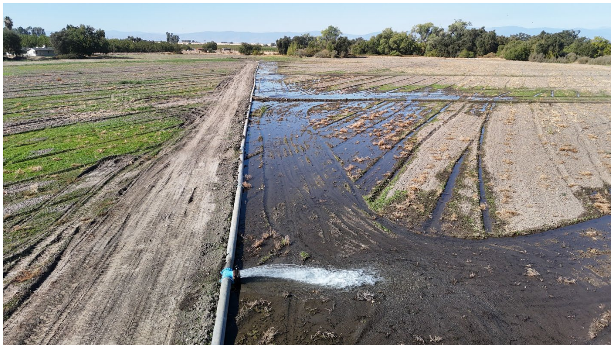
Figure 3-2. Pilot Test #2 Basin Showing Pipeline and Outlets
