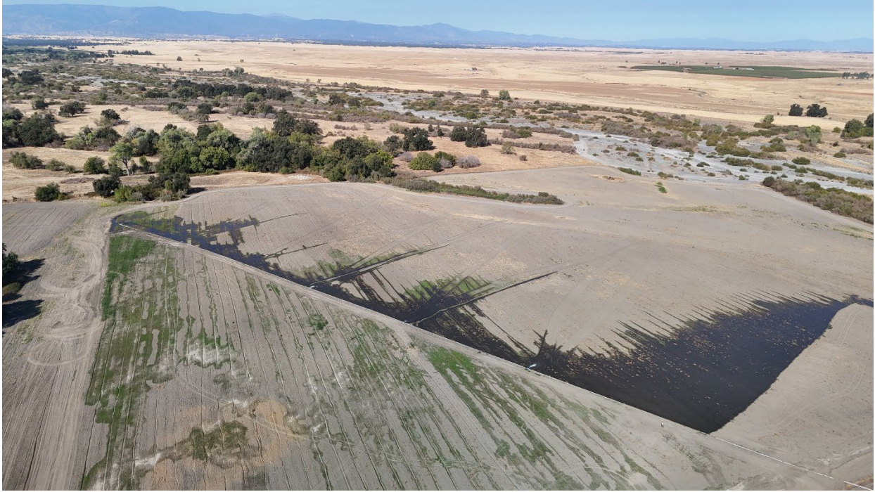
Figure 3-1. Pilot Test #2 Basin Aerial View Looking Northwest
