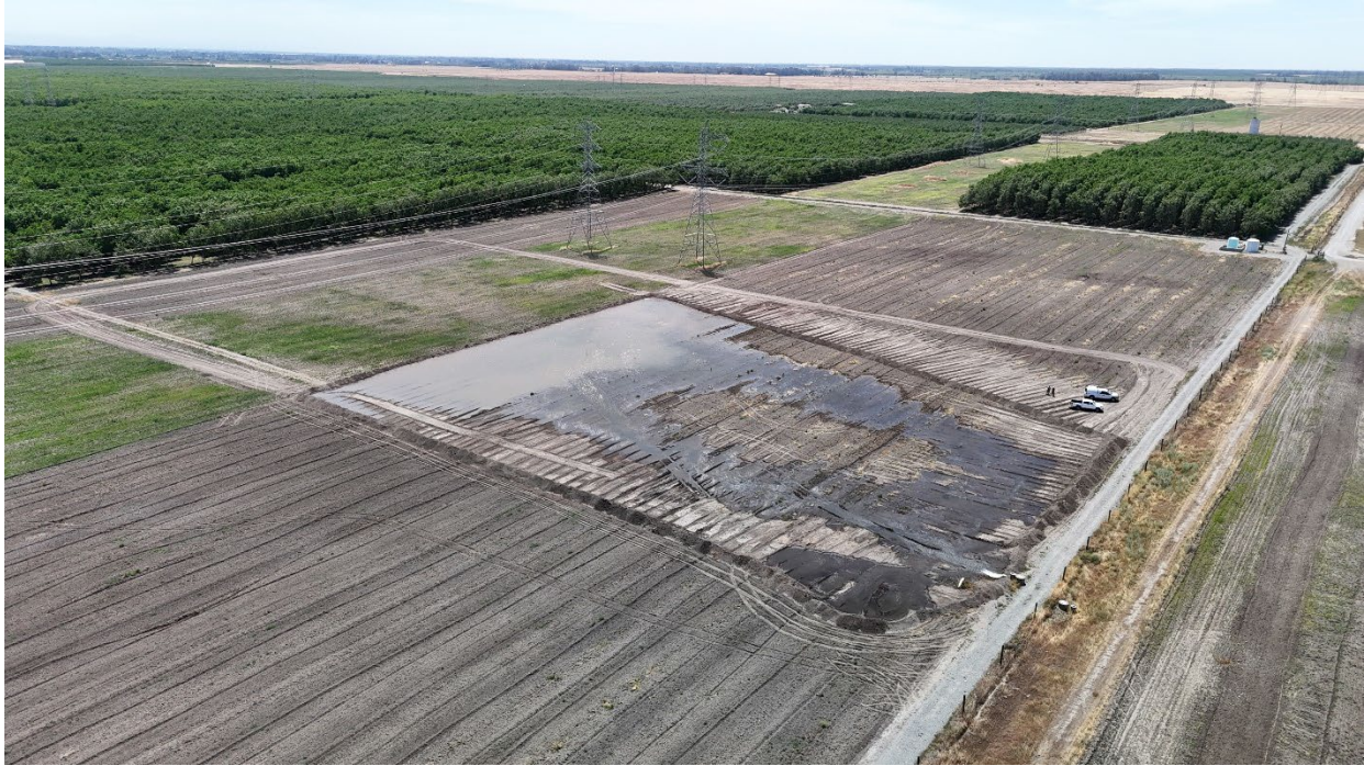
Figure 2-1. Pilot Test #1 Basin Aerial View Looking Southeast
