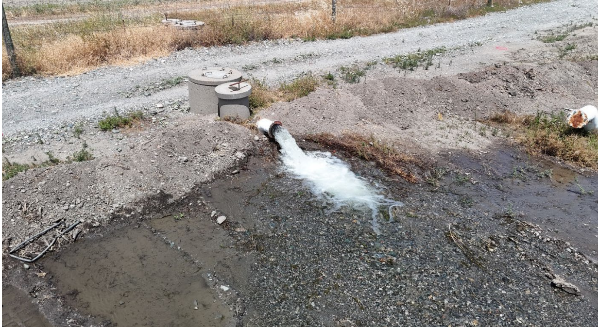
Figure 2-2. CWD Irrigation Infrastructure and Water Flowing into the Basin
