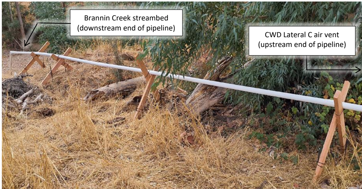
Figure 4. Temporary pipeline and support structure spanning the distance between the CWD Lateral C air vent and Brannin Creek streambed (approximately 60 feet (FT) of 2" PVC pipe).
