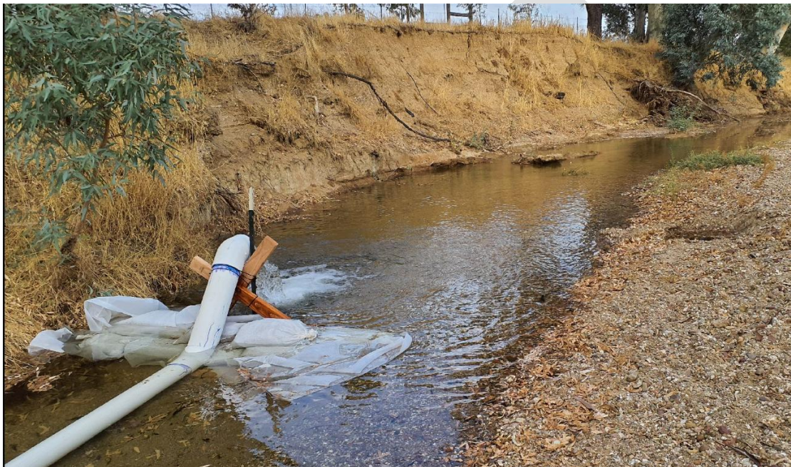
Figure 6. Surface water flow redirected from CWD Lateral C into the Brannin Creek streambed for Instream Recharge Feasibility Study.
