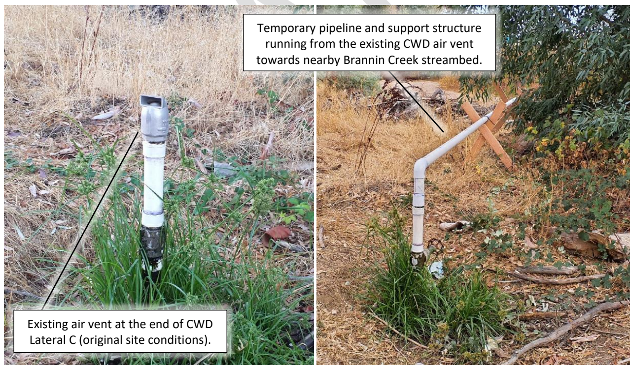
Figure 3. Source of water for Brannin Creek Instream Recharge Feasibility Study, consisting of a temporary pipeline retrofitted to connect to existing infrastructure (an air vent located at the end of CWD Lateral C).
