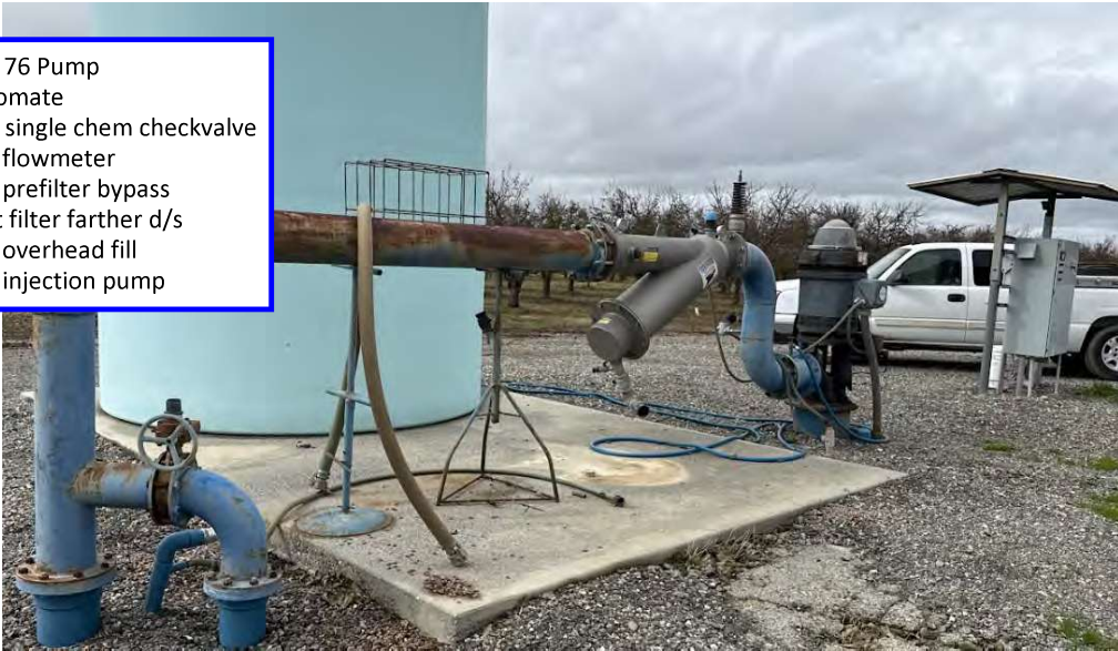
Top Pump - Automate - add flowmeter - add prefilter bypass - add injection pump
