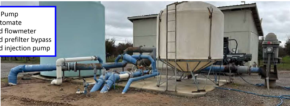
West 100 Pump - Automate - add flowmeter - add injection pump
