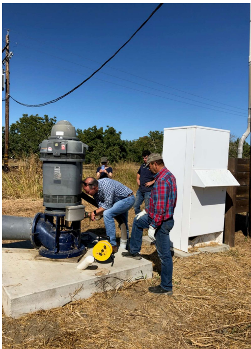
Figure 13. Installing a pressure transducer in a well head.
