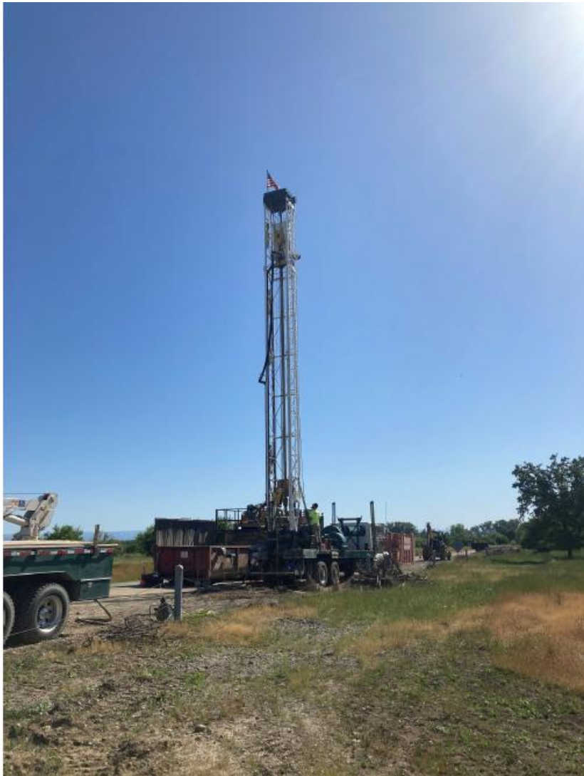
Corning Subbasin-During Construction
